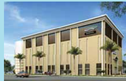
Motor City - District Cooling Plants
