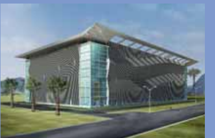
Nad El Sheba - Central Cooling Plant
