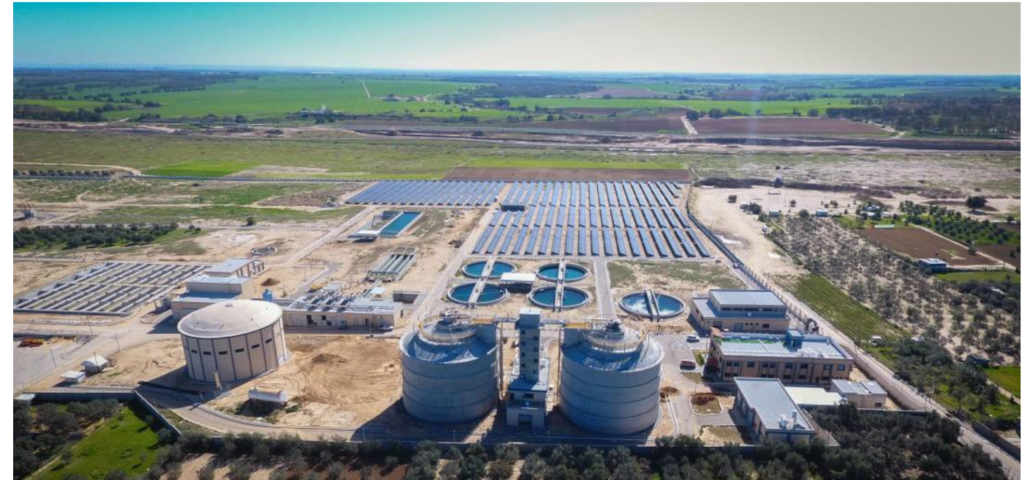
Wastewater Treatment Plant in Gaza
